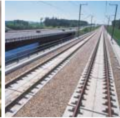
Slab track system Bögl at the ICE-high-speed-line Nuremberg–Ingolstadt
