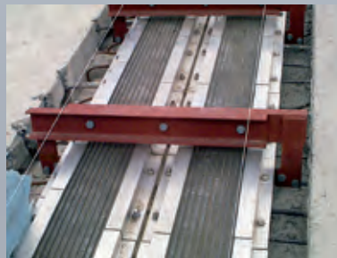
Conventional installation method, that is the prefabricated DB 160 expansion joint is lowered into an existing blockout and then concreted.
