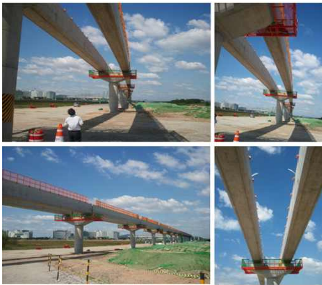
Figure 7. Guideways under Construction
