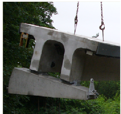
Figure 12: Mounting of fully equipped girder
