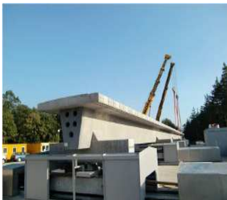
Figure 14: Prototype of flexible concrete switch
