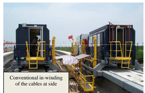
Figure 9: In-Winding of cables in Shanghai
