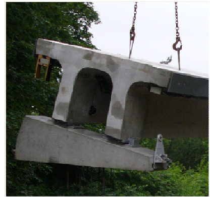
Figure 12: Mounting of fully equipped girder
