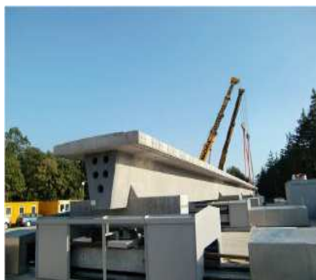
Figure 14: Prototype of flexible concrete switch
