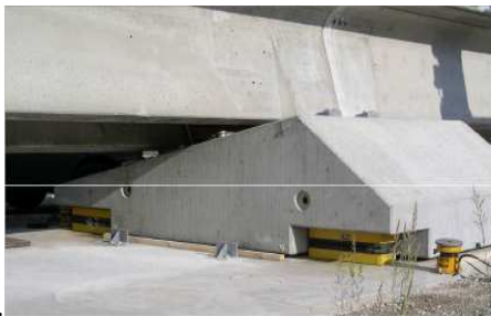
Figure 15: Mass-spring-system with elastomeric bearing
