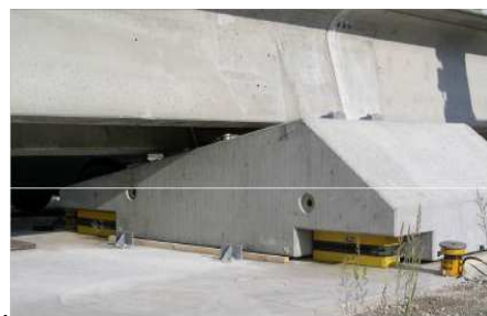
Figure 15: Mass-spring-system with elastomeric bearing
