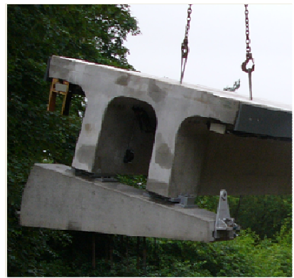
Figure 12: Mounting of fully equipped girder
