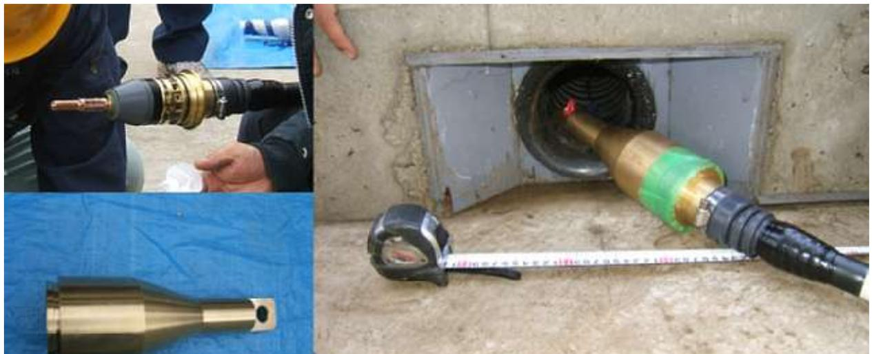
Figure 12. Terminal part protective cover and the use situation
