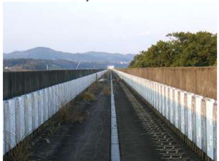
Figure 2. Section of side wall levitation
