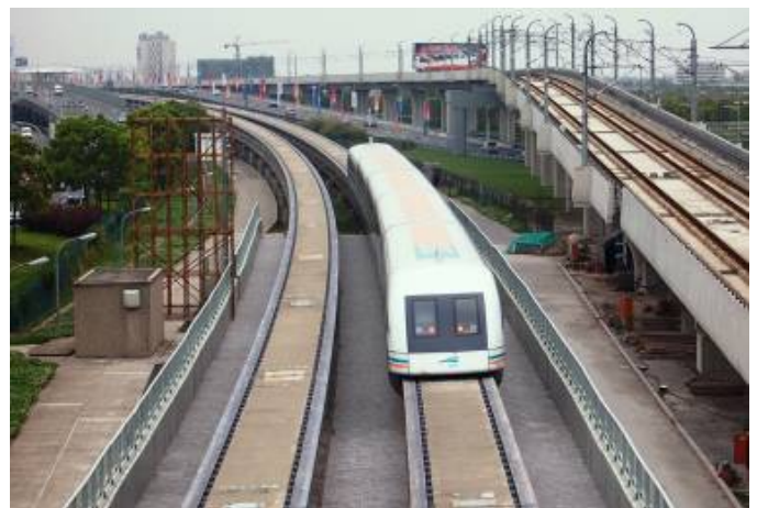
Figure 7 Simulation test of new type of on-bridge girder structure on SMDL.
