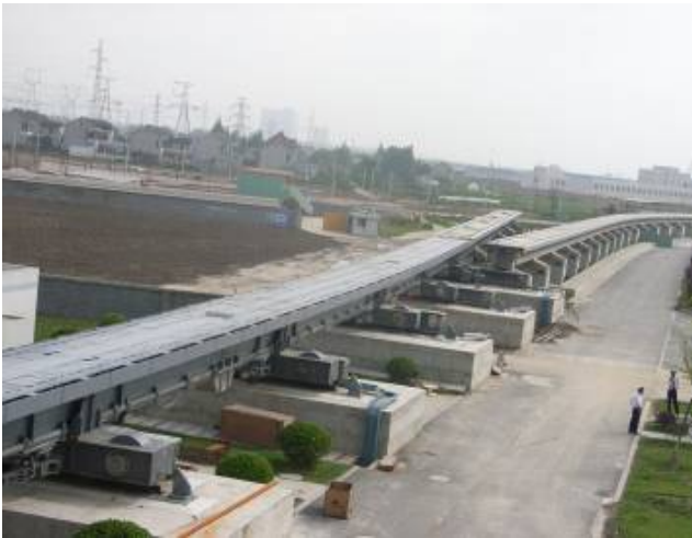
Figure 5. Newly developed low speed switch under test.
