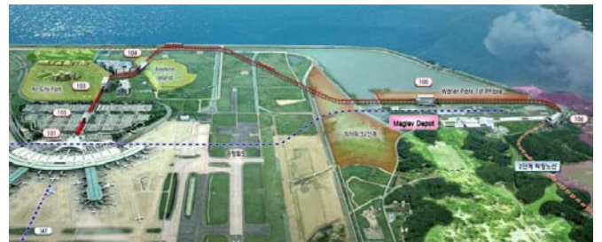
Figure 1. Commercial maglev line in Incheon International Airport, Incheon, South Korea.
