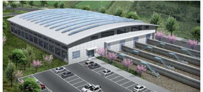
Figure 4. An air view of Inspection Shed Building
