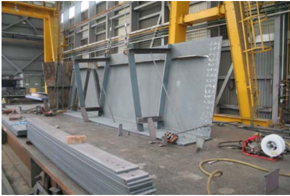
Figure 12. Manufacturing the trapezoidal open steel box girder segment
