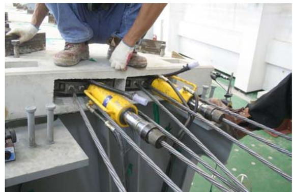
Figure 17. Introduction of prestressing forces to the decks
