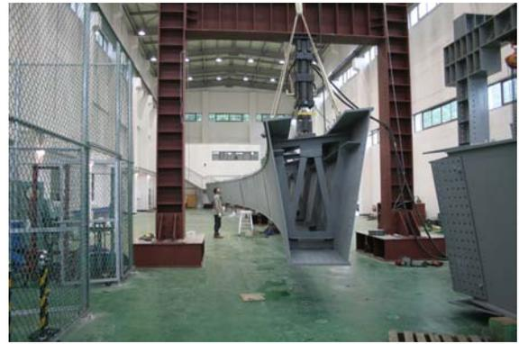
Figure 14. View during installation of main girder segments
