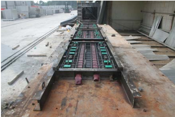
Figure 8. 3 Steel forms and arrangement of reinforcement bar
