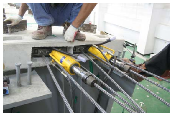
Figure 17. Introduction of prestressing forces to the decks
