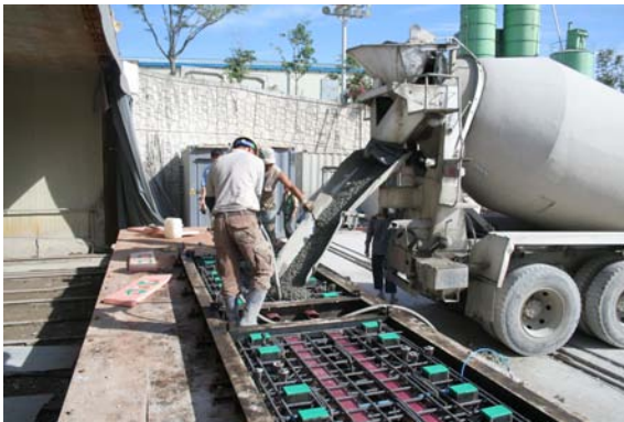
Figure 9. Casting of concrete into steel form
