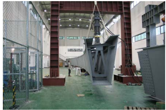
Figure 14. View during installation of main girder segments
