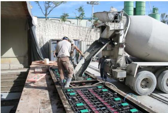
Figure 9. Casting of concrete into steel form
