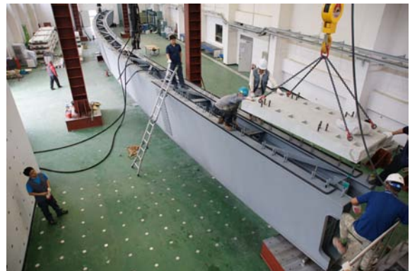
Figure 16. Placement of precast decks onto the main girder
