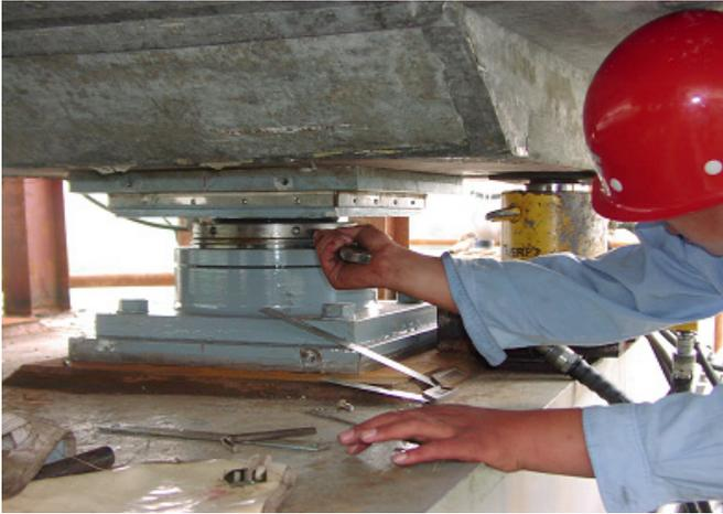
Figure 13: Adjustment of bearing
