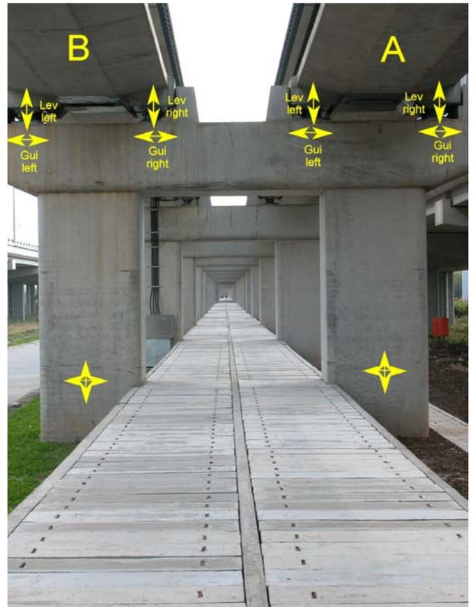
Figure 9: Measurement channels relatively to the guideway
