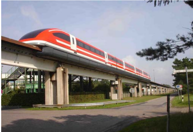
Fig. 11: Installation of prototypes at the TVE.
