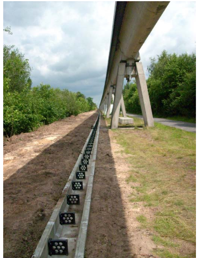
Figure 5: TVE track section for testing of the new cable clamps
