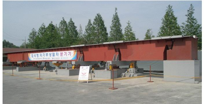
Figure 5. 3 way segmented maglev switch
