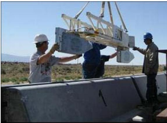
Figure 9. Sled/magnet shown being installed in guideway
