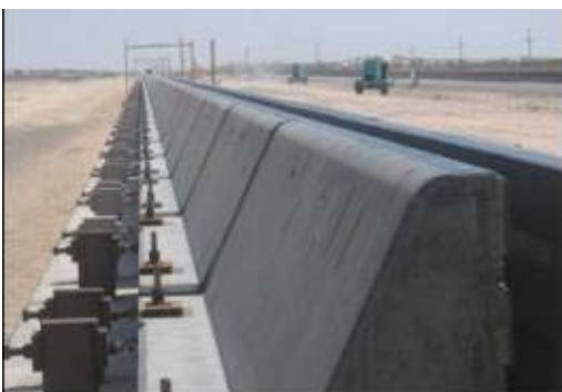
Figure 5. Guideway beams looking south.
