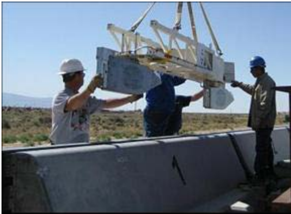
Figure 9. Sled/magnet shown being installed in guideway
