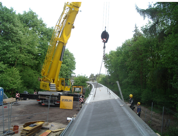
Picture 12: Installation of the guideway slab in the “south-loop”-section
