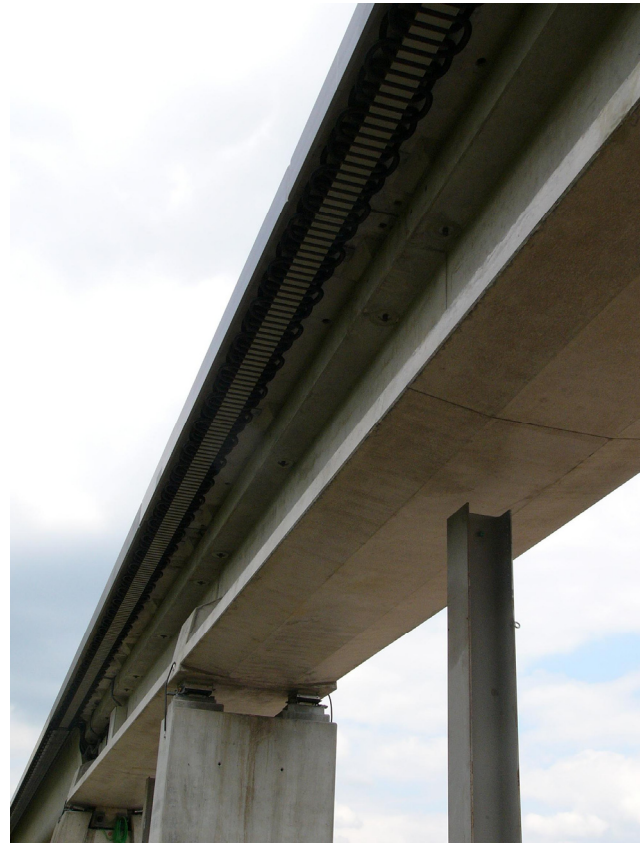
Picture 13: MSB-Track-2010, mounted on a precast beam on the TVE
