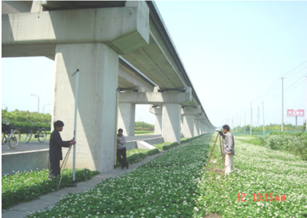
Figure 1: Measurement beside the track in daytime
