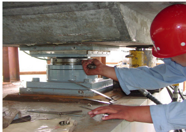
Figure 3: Bearing adjustment
