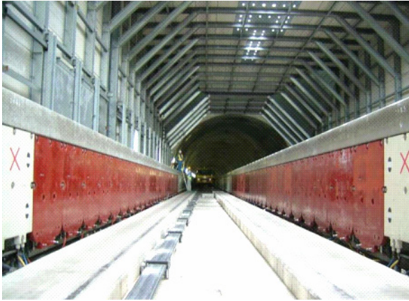
Figure 5: 120-degree pitch levitation coils.
