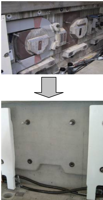
Fig. 6: Side-wall shape of Integrated-type Coils
