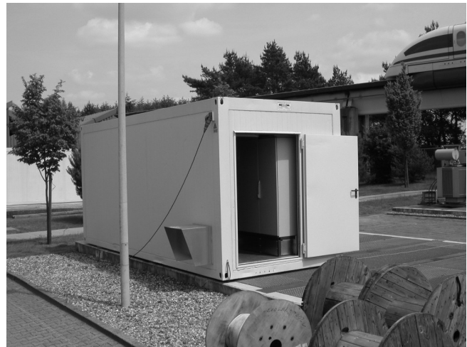
Figure 6: Induction loop at the guideway (left) and container with power supply near the maintenance hall (right) for the IPS ® system test on the TVE.
