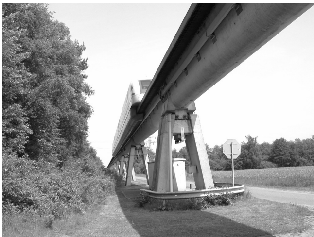
Figure 6: Induction loop at the guideway (left) and container with power supply near the maintenance hall (right) for the IPS ® system test on the TVE.
