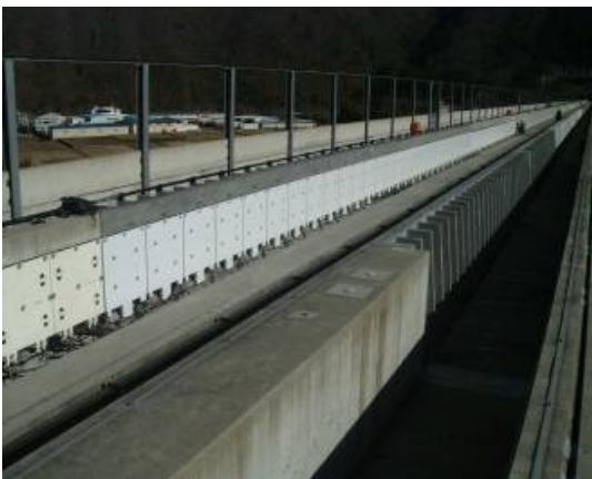
Figure 3: Lightweight UFC guideway sidewall
