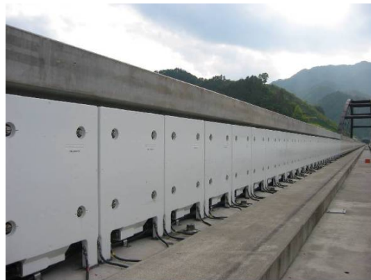
Figure 4: Integrated type coils
