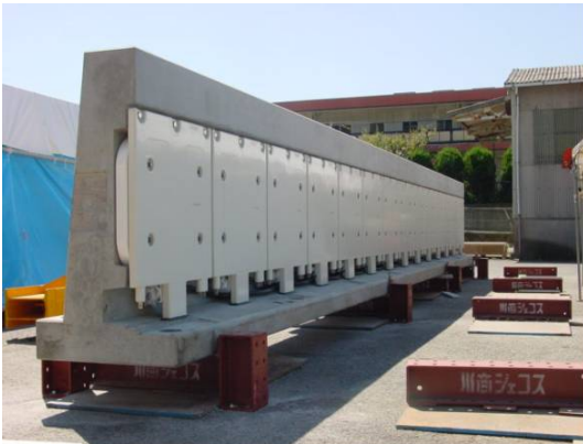
Figure 2: Self-standing guideway sidewall
