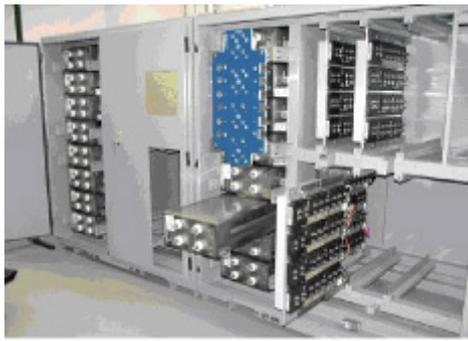
Figure 7: IGBT-based Advanced Power Electronic Converter System
