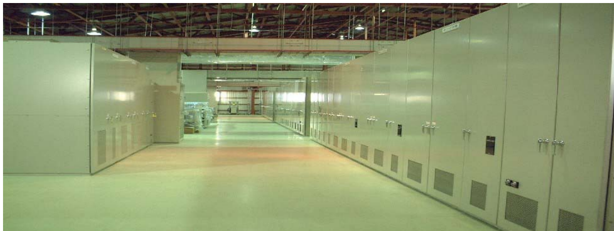
Fig.3 New IEGT inverter(left) and former GTO inverter(right)
