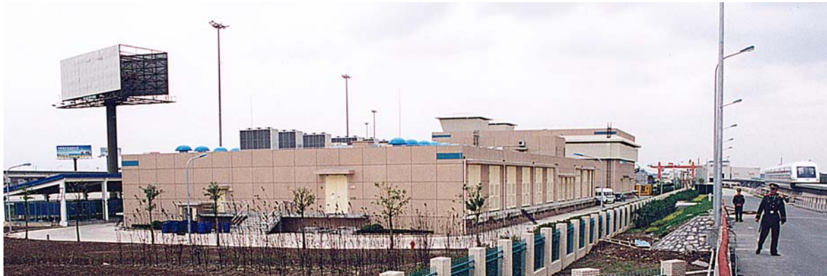
Fig. 2: Power Substation 2 (Pudong) of the Shanghai Transrapid
