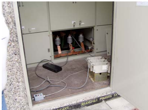
Fig. 8: Earth fault protection test at the Shanghai Transrapid Project
