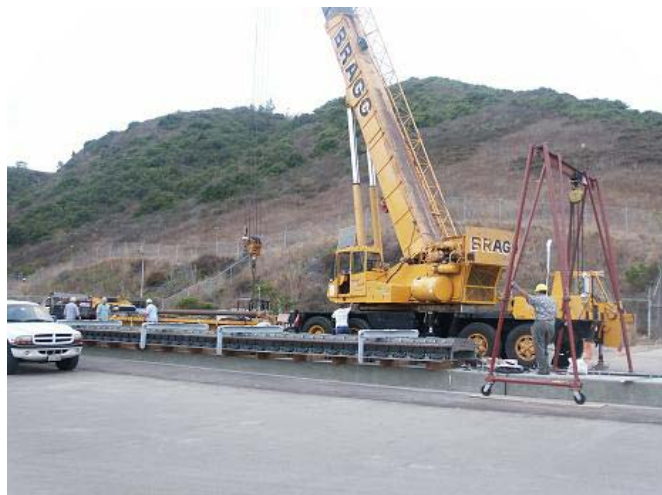
Figure 4. Completed 120-m test track foundation, and first 15-m guideway weldment (left). Right picture shows completed guideway module ready for turning over.
