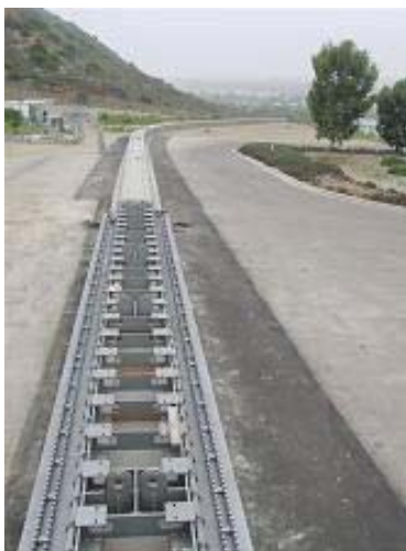
Figure 4. Completed 120-m test track foundation, and first 15-m guideway weldment (left). Right picture shows completed guideway module ready for turning over.
