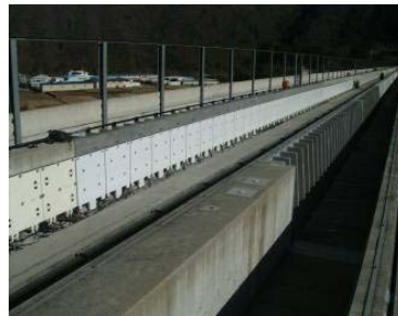
Fig. 6 Lightweight RPC sidewalls
