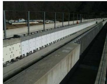
Fig. 6 Lightweight RPC sidewalls
