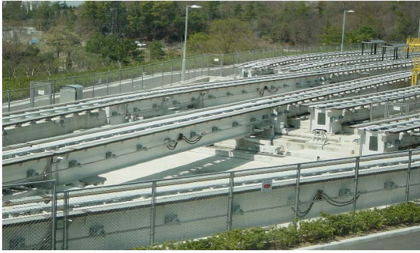
Photo-2 The Segmented type switch
