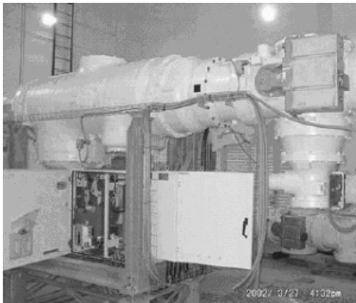
Figure 10: Gas insulated switchgear in 110 kV substation Long Yang Road
