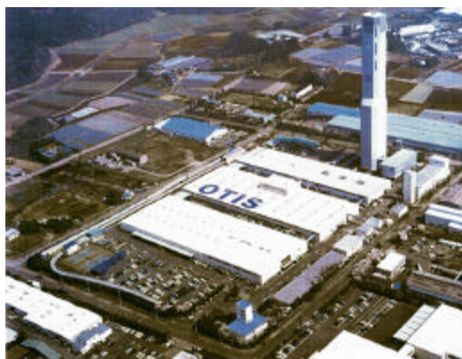
Figure 2. Test track in Shibayama factory, Chiba Pref.
