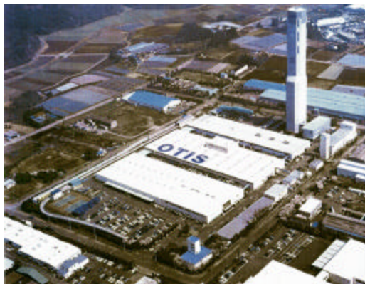
Figure 2. Test track in Shibayama factory, Chiba Pref.
