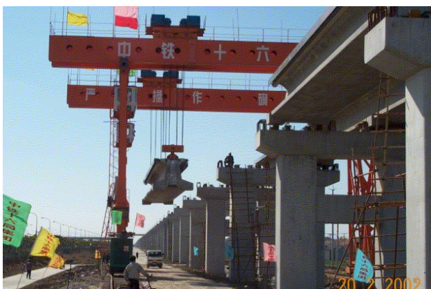
Fig. 16: Mounting of Hybrid Guideway Girders
