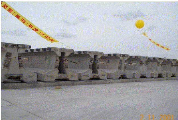
Fig. 15: Type I girders on the storage yard
