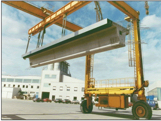
Fig. 9: Prototype girder at the site
