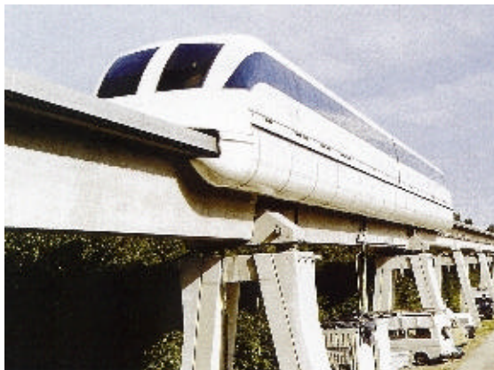
Fig. 11: Transrapid TR07 on the Hybrid Girder at TVE
