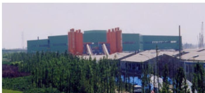
The production hall has measurements of the outline in a larger way 100 x 200 m and a height of approx. 12 - 14 m. In the hall all trades are put, that are used for the production of the prestressed concrete box girder as main structure. In front of the hall the concrete plant was built up. The 2<sup>nd</sup> third of the ground is needed as a stor-
